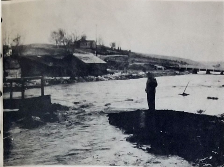
LOU LINDNER watches as water gushes by footbridge on Franklin Street. The east approach to the bridge had been ripped out after the flood water in Esquatzel ditch threatened to spill over and inundate the downtown business section.
